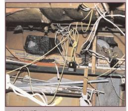
Modifications to electrical wiring can create a fire hazard.
