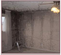
Moisture from grow ops can cause structural damage.
